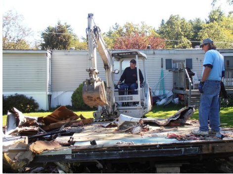
Brian B. works the mini excavator while Mike looks on.
